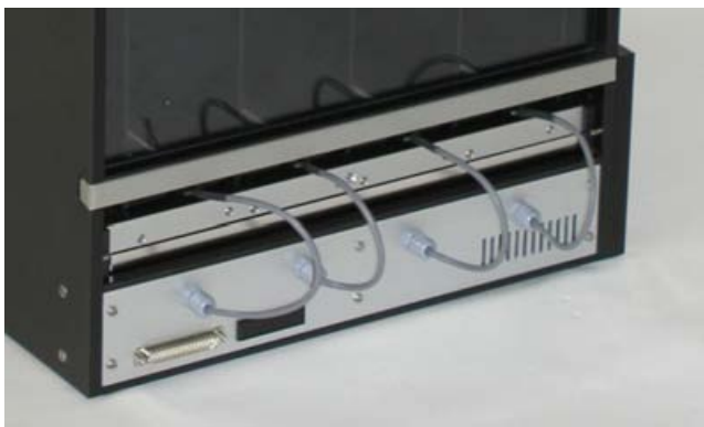
Shocker cables leading to the floor grids (backside)
